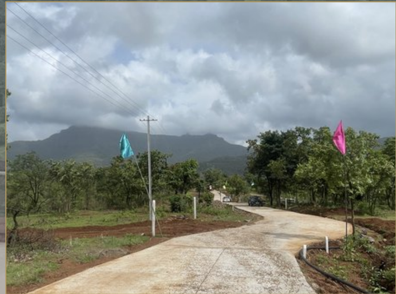
SITE PHOTOGRAPH · INTERNAL ROAD
